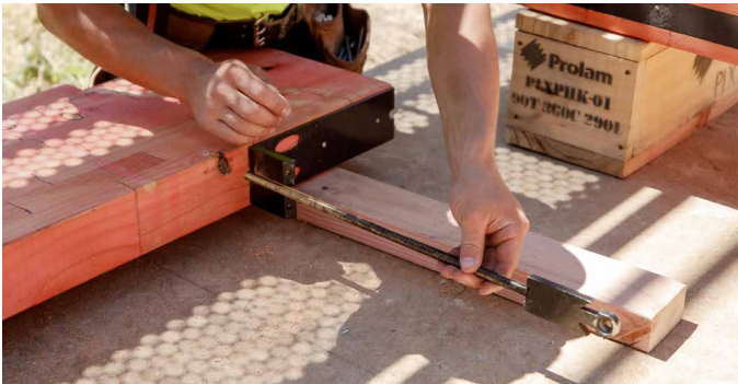
3. Install bottom dovetail rod into each column.
