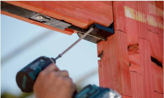
3. Square up the portal then add 4x VGZ 7x200 uplift screws into the L-Brackets at 45 degrees.
