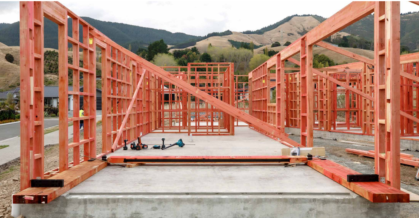
1. Lay down columns and lintel (ensure lintel is the correct way up) in place on the ground.
