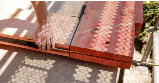
4. Sit lintel into place on L-brackets and add the top dovetail rods.
