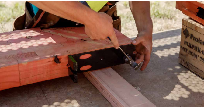
2. Nail the L-Brackets to the unrebated side of each column.
